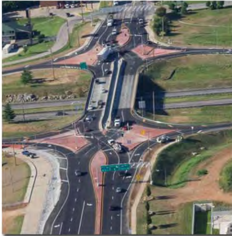
The First DDI in the U.S. located in Springfield, MO at the interchange of I-44 and Route 13
