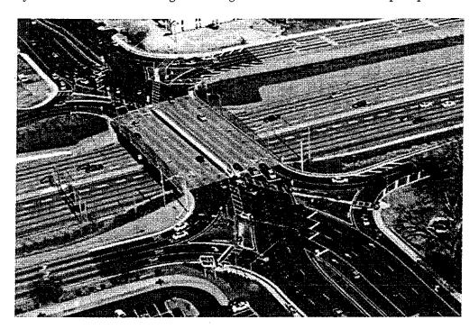
After crossover, construction will continue on the center median and pedestrian facilities, while crews will finalize the signals, interchange lighting and pavement markings. The project is expected to be substantially complete in September, with landscaping to begin in the fall. Once the project is complete, the bridge at Pleasant Hill Road and I-85 will be Gwinnett County's first DDI and the second in Georgia.
